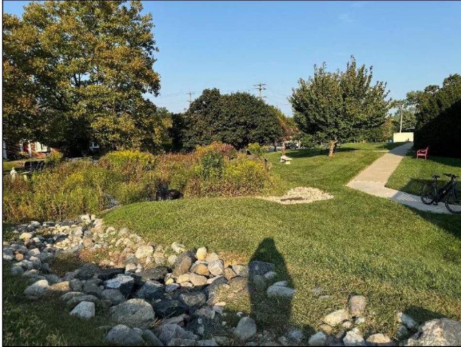
Photo 3: Landscaping and Stormwater Management Facility/Rain Garden
