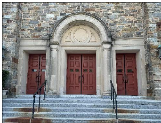
Photo 9: Exterior Windows and Doors
