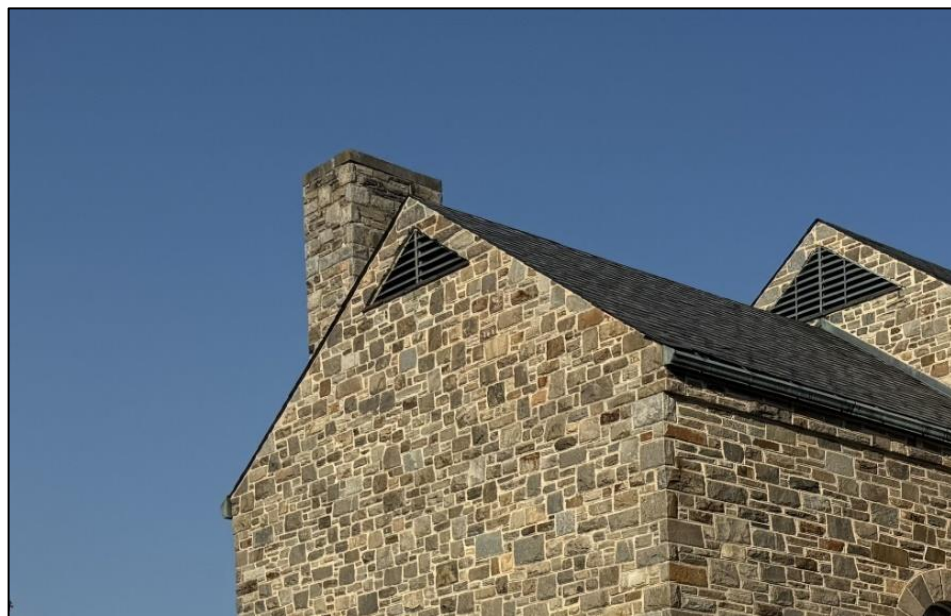
Photo 8: Roofing and Envelope System
